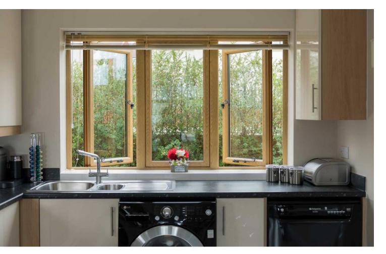
When it comes to the upkeep of moving parts, at TWS we are confident that the regular maintenance and lubrication of your windows and doors' moving parts will help prolong their longevity (we recommend this is done in the spring and autumn). Hinges and handles will require lubrication with silicone spray to keep them working at their best. On the contrary to popular belief, do not use WD40 as it has the opposite effect by ceasing up the rubbers 'grease' and making it even harder to slide.
